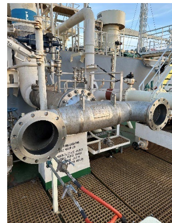
Figure 12 Y-Piece installed on FSRU ALEXANDROUPOLIS
