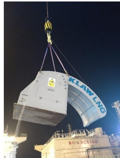
Figure 36 Transfer of Saddles
