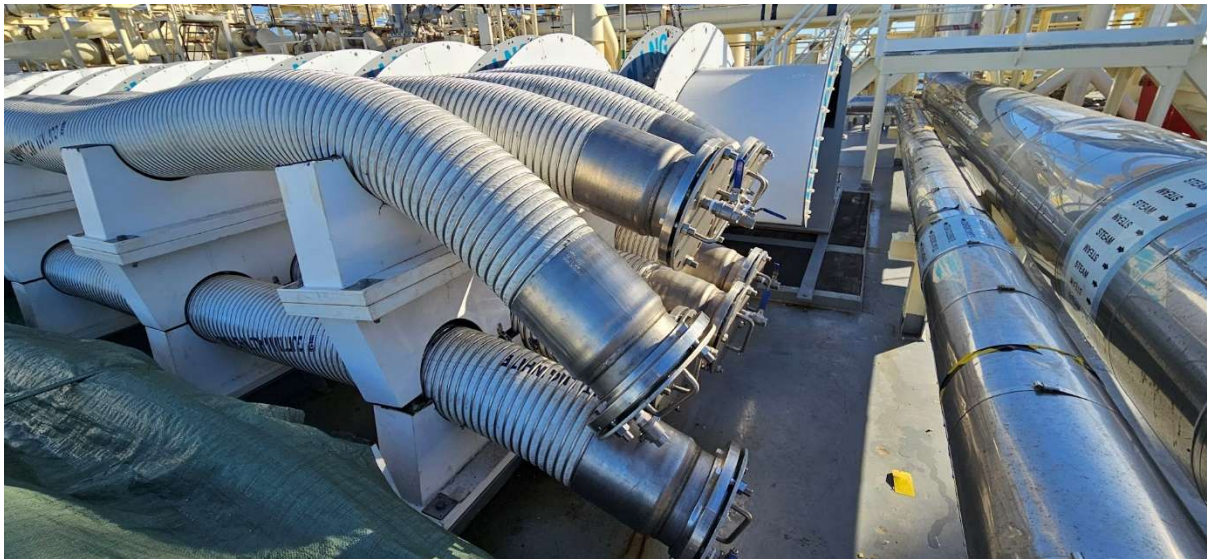
Figure 8 Gutteling Multi-LNG White Hose
